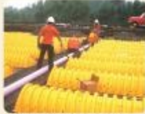
Installation of the infiltration chambers prior to re-seeding the grassy field.
