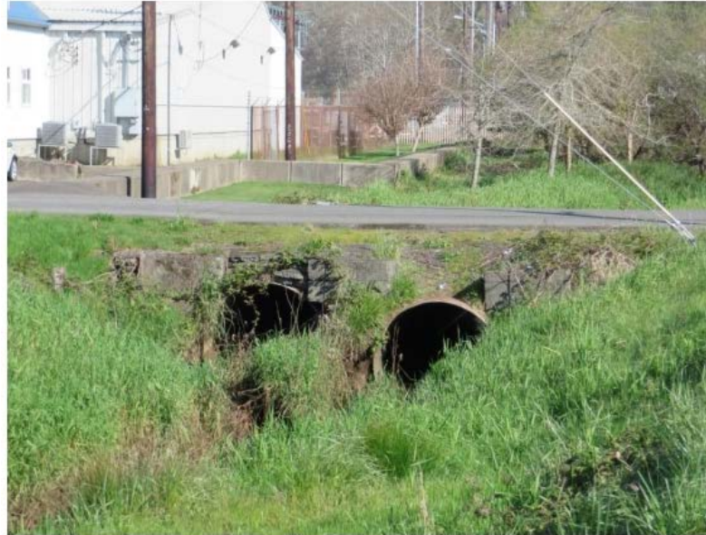
FRY CREEK - CULVERT CONSTRICTIONS
