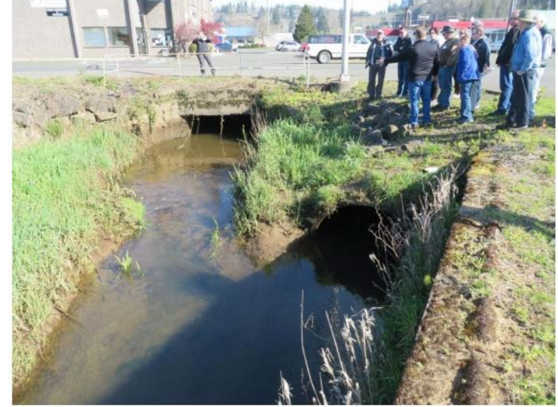
FRY CREEK - CULVERT CONSTRICTIONS
