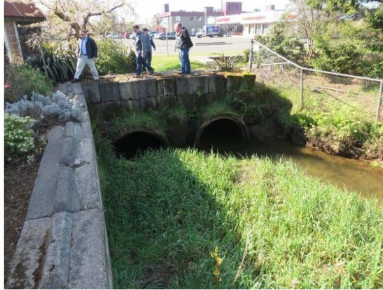
FRY CREEK - CULVERT CONSTRICTIONS
